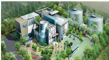
오폐수처리장 WASTEWATER TREATMENT PLANT
